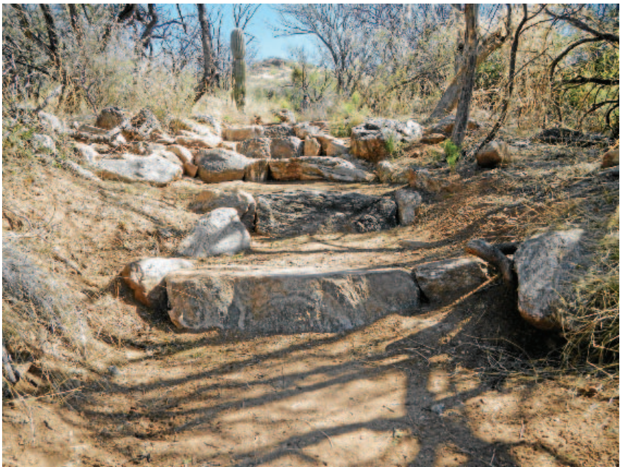
The magic of the check dams is hidden beneath the surface. Crews transport, dig holes for, bury and perfectly set large rocks to create the dam that holds the bed in place.
